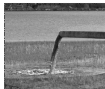
Sewage being piped into a river
