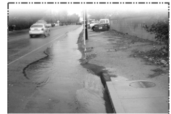
Storm water drain
