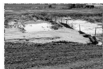
Silt fences used to prevent soil erosion
